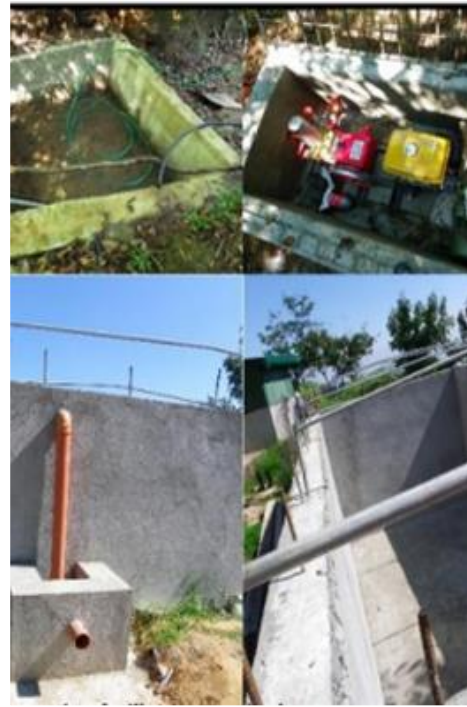
Water Harvesting Facility
