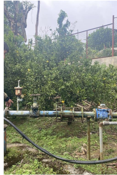
Water Harvesting Facility
