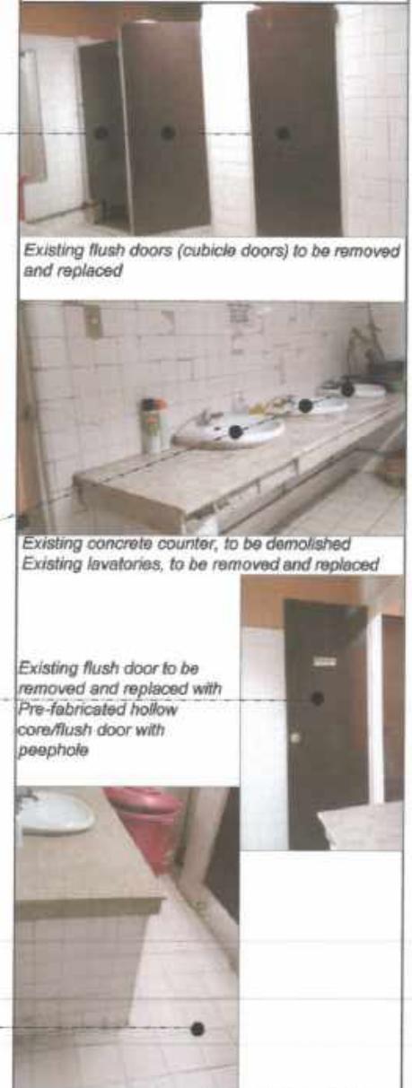
Existing floor tiles, to be removed and replaced with 40mm x 40mm porcelain textured non-slip floor tiles
