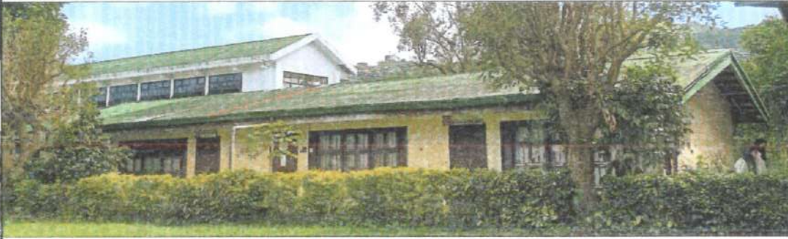
Existing corrugated roofing sheets to be removed and replaced
