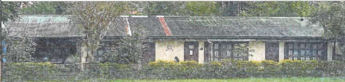
Existing wood awning window to be removed and replaced with pre-fabricated steel awning window with grills Existing wood panel door to be removed and replaced with pre-fabricated steel door Center door to be removed and to be covered with chb ; plaster and paint finished
