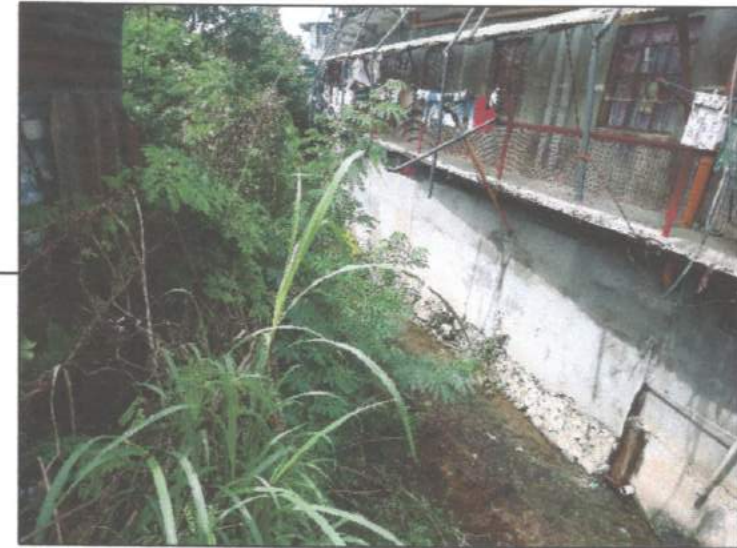
START OF PROJECT
